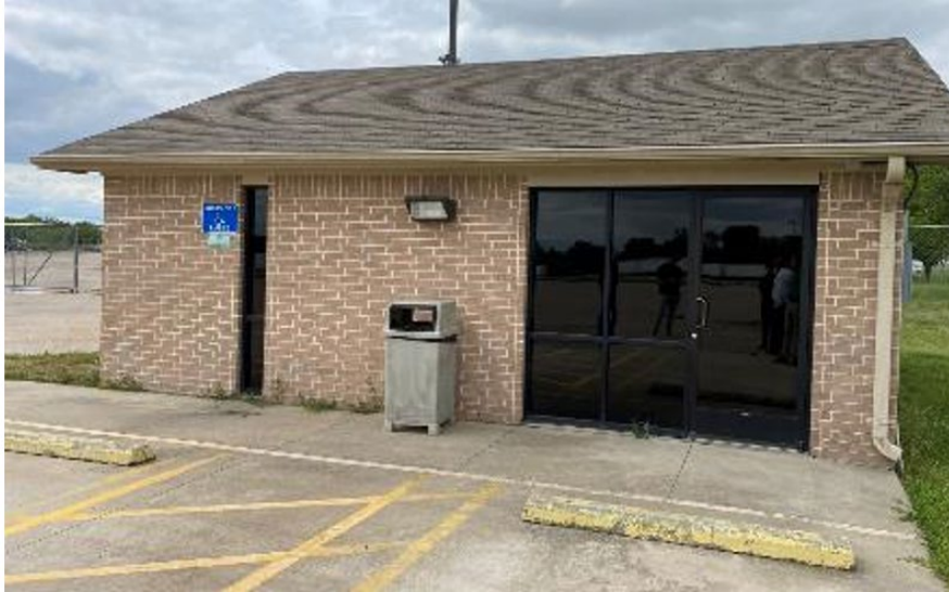
700 SF MASONRY DISPATCH
